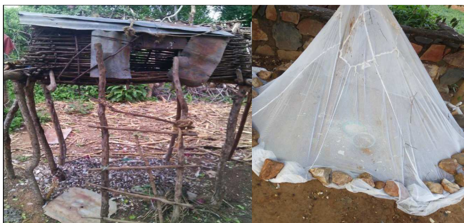
Fig. 4: Common poultry house present in the study area; Source: Photo from field farm at Nyagatare Sector
