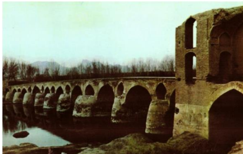
Fig. 2: The Shahrestan Bridge Source: Ayatollah-Zadeh-Shirazi, 2013, p. 33
