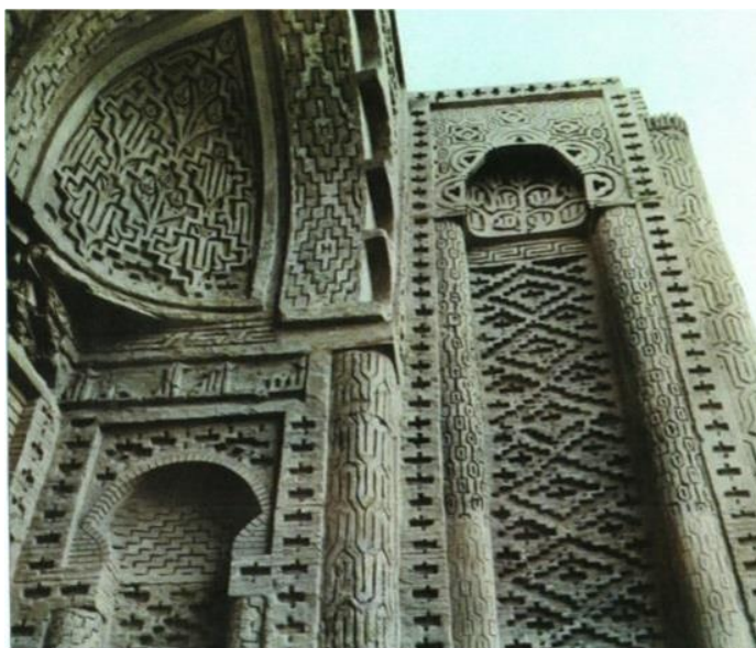
Fig. 6: Entrance facade of the Jorjir Grand Mosque, 4th Century A.H. Source: Ayatollah-Zadeh-Shirazi, 2013, p. 41
