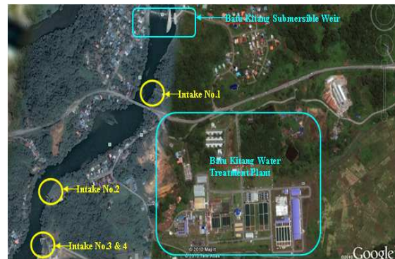
Fig. 3: Location of raw water intakes and submersible weir at BKWTP
