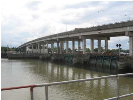
Fig. 6: Barrage radial gates and bridge
